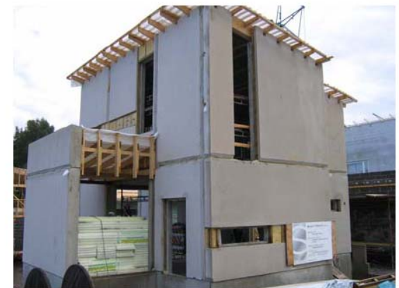
Fig 11. Plastered precast sandwich panels erected.
