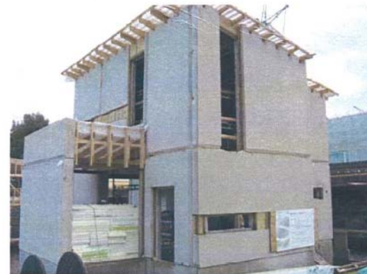
Fig 11. Plastered precast sandwich panels erected.
