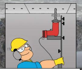
INSPECT AND OPEN DRAINAGE HOLES AFTER JOINT GROUTING. DRILL MORE HOLES IF NECESSARY.
