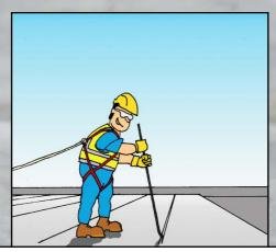
STEER THE SLAB INTO PLACE WITH AN INSTALLATION BAR. BE CAREFUL OF SLIPPERINESS IN THE WINTER.
