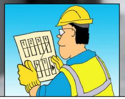
DRAW UP AN INSTALLATION PLAN WELL IN ADVANCE AND AGREE ON THE ORDER OF THE DELIVERY OF THE SLABS. SELECT A LIFTING DEVICE THAT IS SUITABLE FOR THE SITE CONDITIONS AND THE WEIGHT OF THE HOLLOW-CORE SLABS.
