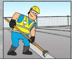
REMOVE ANY EXCESS GROUT. ALSO CLEAN THE SOFFIT OF THE SLAB. CARRY OUT PROTECTION AND CURING ACCORDING TO THE CONDITIONS.
