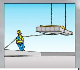
IF NEEDED, ATTACH A ROPE TO THE SLAB THAT IS BEING LIFTED IN ORDER TO ASSIST IN DIRECTING IT.
