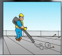
CLEAN SNOW, ICE AND DEBRIS FROM THE JOINTS. INSPECT THE VOID PLUGS AND CARRY OUT FORMWORK FOR THE JOINTS.
