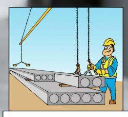
ALWAYS LIFT BY USING LIFTING LOOPS OR ANCHORS, IF AWAILABLE IN THE SLAB.
