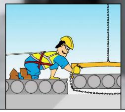
DO NOT DETACH THE SAFETY CHAIN UNTIL THE SLAB IS NO MORE THAN 100 MM ABOVE THE SUPPORT.
