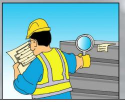
COMPARE EACH SLAB WITH THE PLAN. INSPECT THE SLAB LABELS IN THE LEVEL DRAWINGS, THE SUPPORTS FOR THE INSTALLATION PHASE, THE LIFTING NECKS, THE NUMBER OF STRANDS, THE LOCATION OF THE DEEP-PLUGS AND THE SLIPPAGE OF THE STRANDS.
