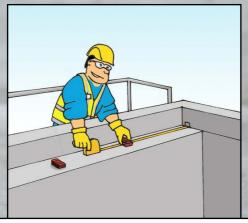
MARK THE LOCATION OF THE SLABS AND SET INSTALLATION SHIMS OR A NEOPRENE BEARING STRIP IN PLACE.
